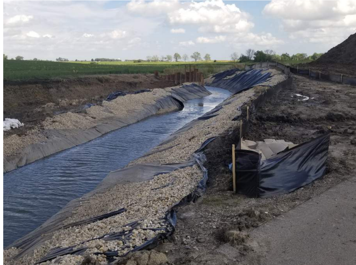
Newly constructed stream diversion channel at Braun Road
